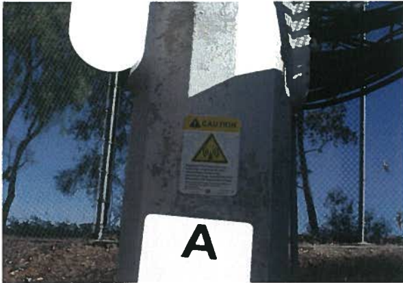
Sector1 Caution sign at the base of the monopole
