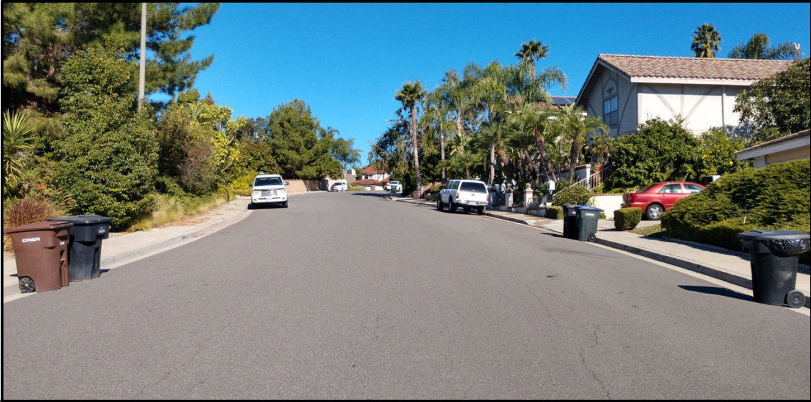
Terra Bella Avenue (Looking Northbound) towards Natama Court
