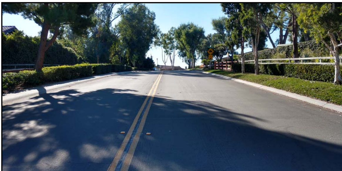
NELLIE GAIL ROAD (Looking Southbound) @ ROCKING HORSE LANE
