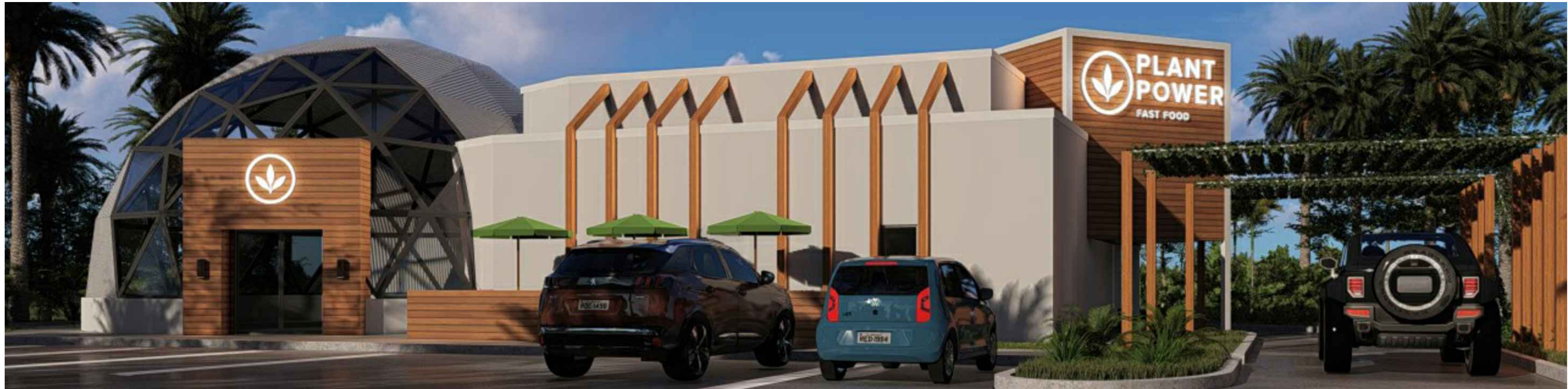
VIEW FROM NORTH
