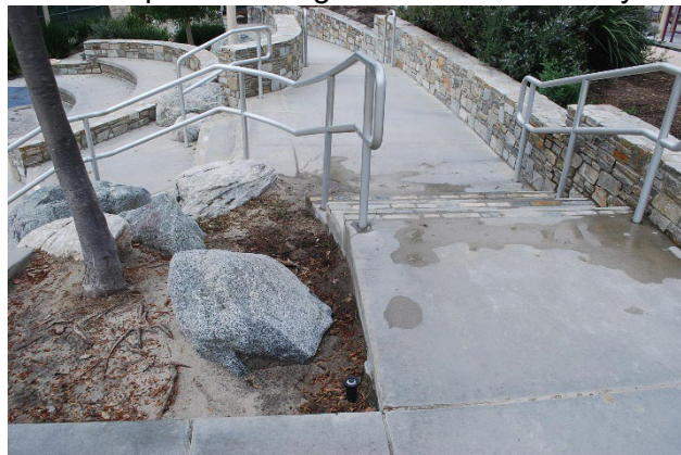
Example Retaining Wall Located Nearby
