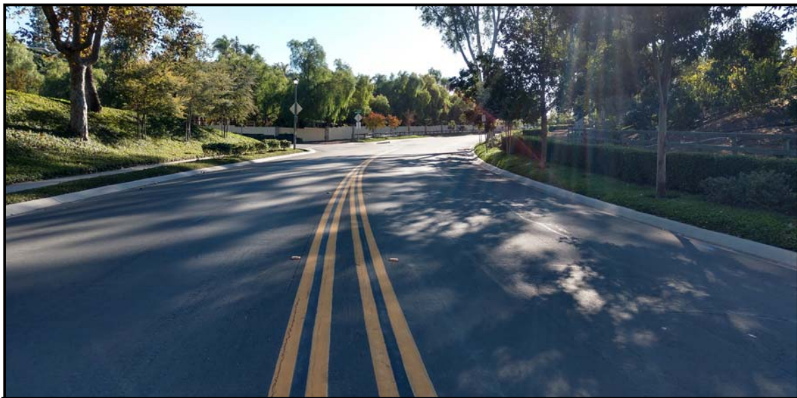
NELLIE GAIL ROAD (Looking Southbound) @ EMPTY SADDLE DRIVE
