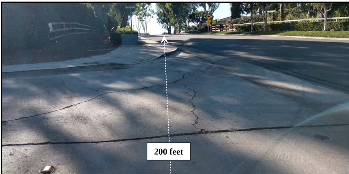
Westbound HIDDEN TRAIL ROAD (Looking South) @ NELLIE GAIL ROAD
