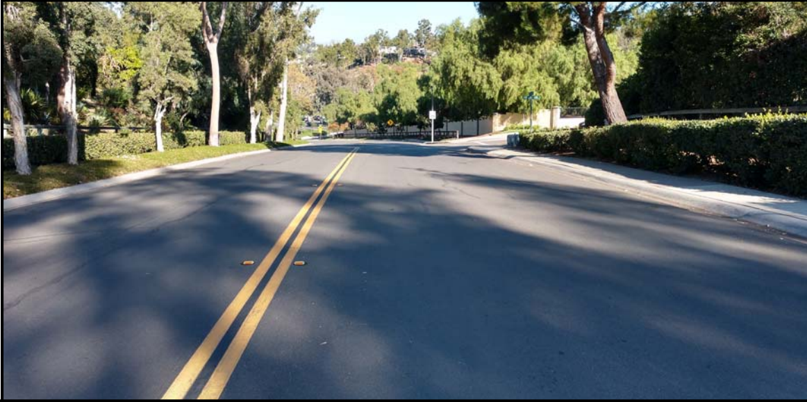
NELLIE GAIL ROAD (Looking Northbound) @ HIDDEN TRAIL ROAD
