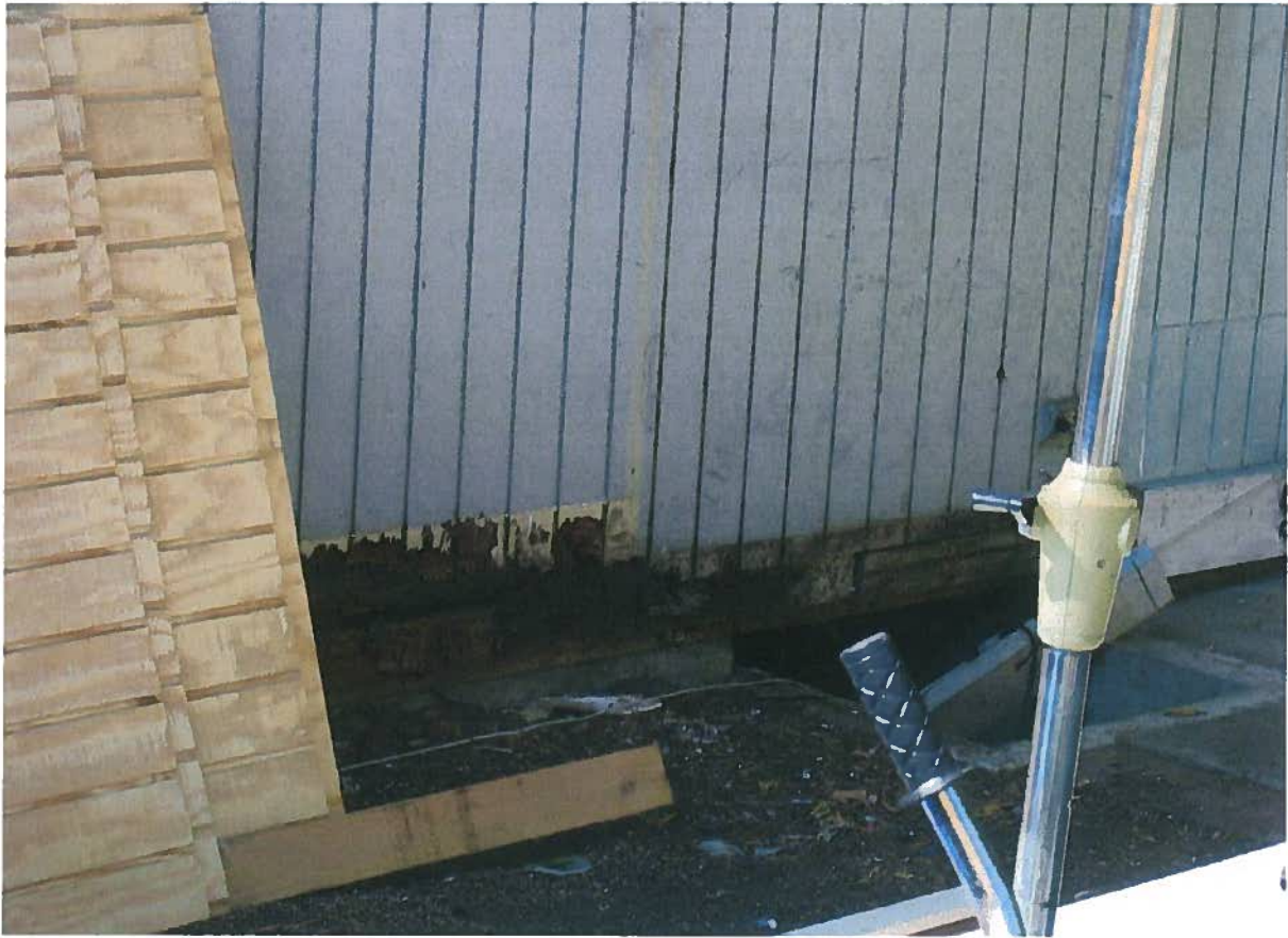
Termite Damage
