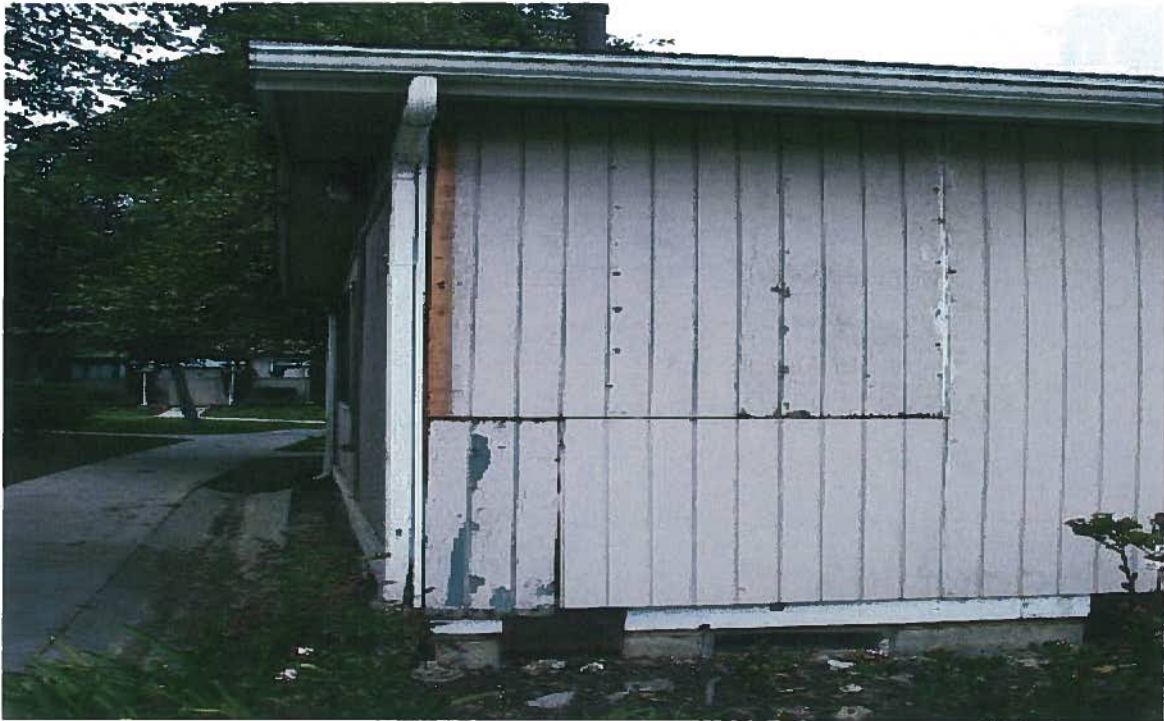
Damaged Siding
