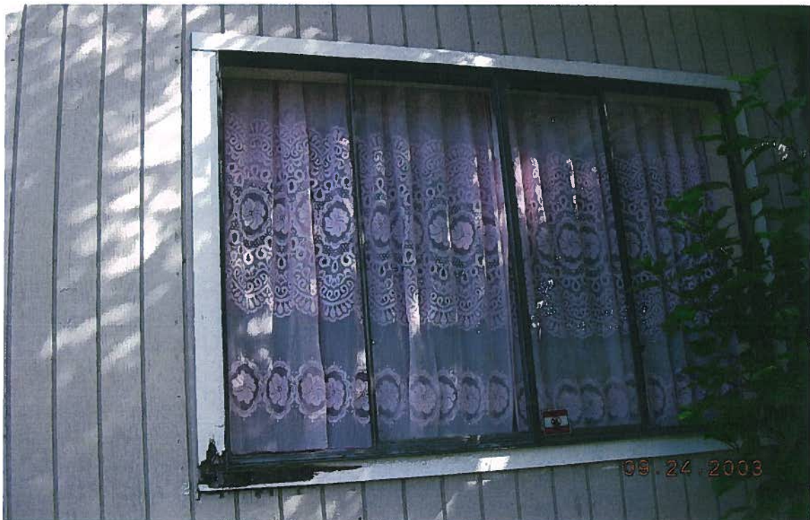
Damaged Siding
