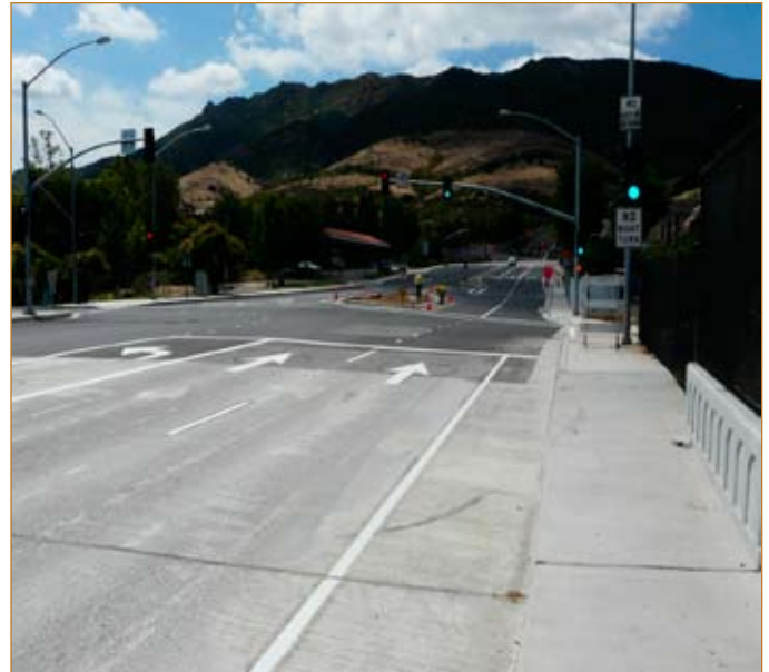
Figure 1. STV designed major intersection improvements, including road widening, for Route 101 at Adobe Reyes Road ▲
