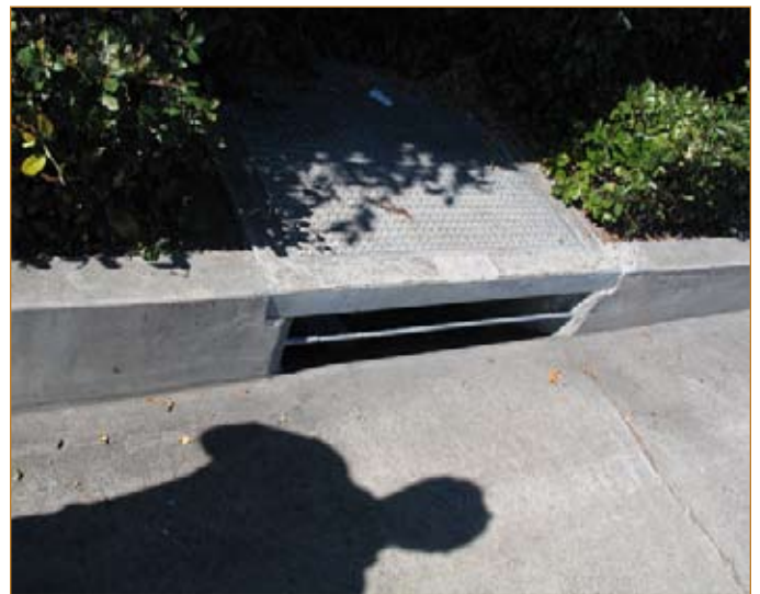
Figure 14. Existing 4-foot inlet along the south-bound lanes ▲
