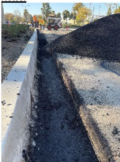
Slot patching in lifts.
