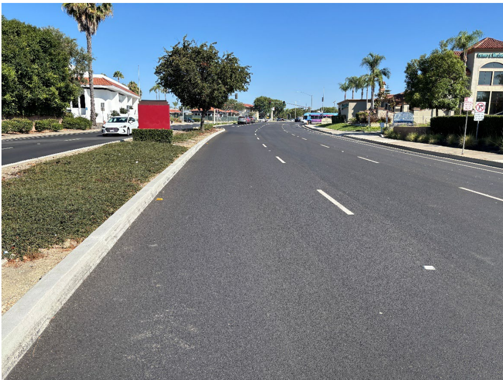
Paseo de Valencia new pavement surface and full height median curbs
