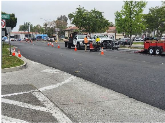
Loop contractor setting up equipment in construction zone for northbound traffic on Paseo Del Valencia.
