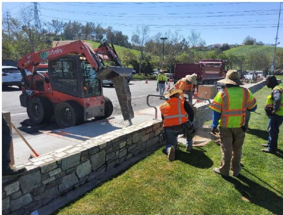
Contractor begins demolition of the stairs into the soccer field at Community Center Park
