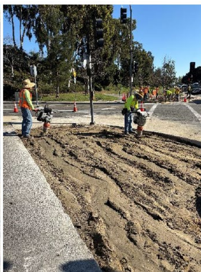
Ramp compaction PDV/Beckenham
