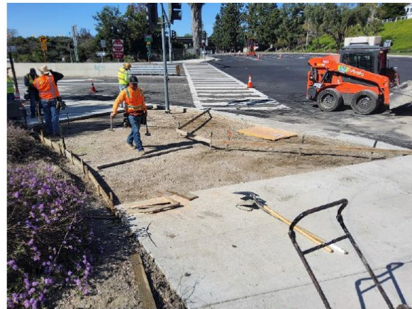
Laborers form ADA ramp at the southeast corner of the intersection of Hwy 73 and La Paz
