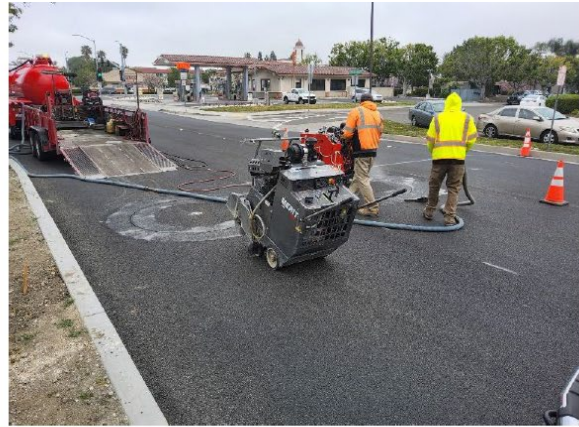
Laborers cut ahead loops for the intersection of El Toro Road and Paseo Del Valencia
