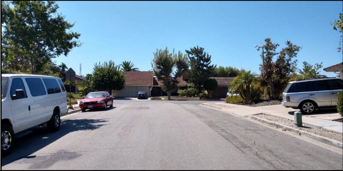
VELASQUEZ ROAD (LOOKING SOUTHBOUND) @ MAWSON DRIVE
