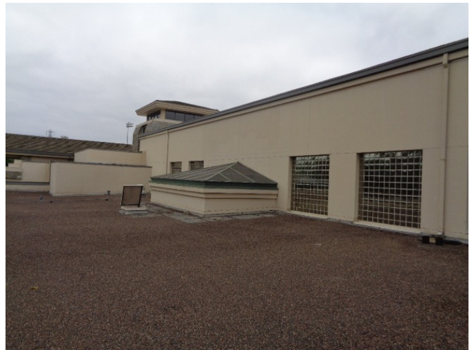
Built up Roof
