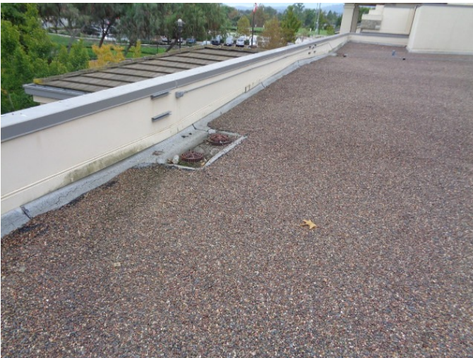
Built up Roof
