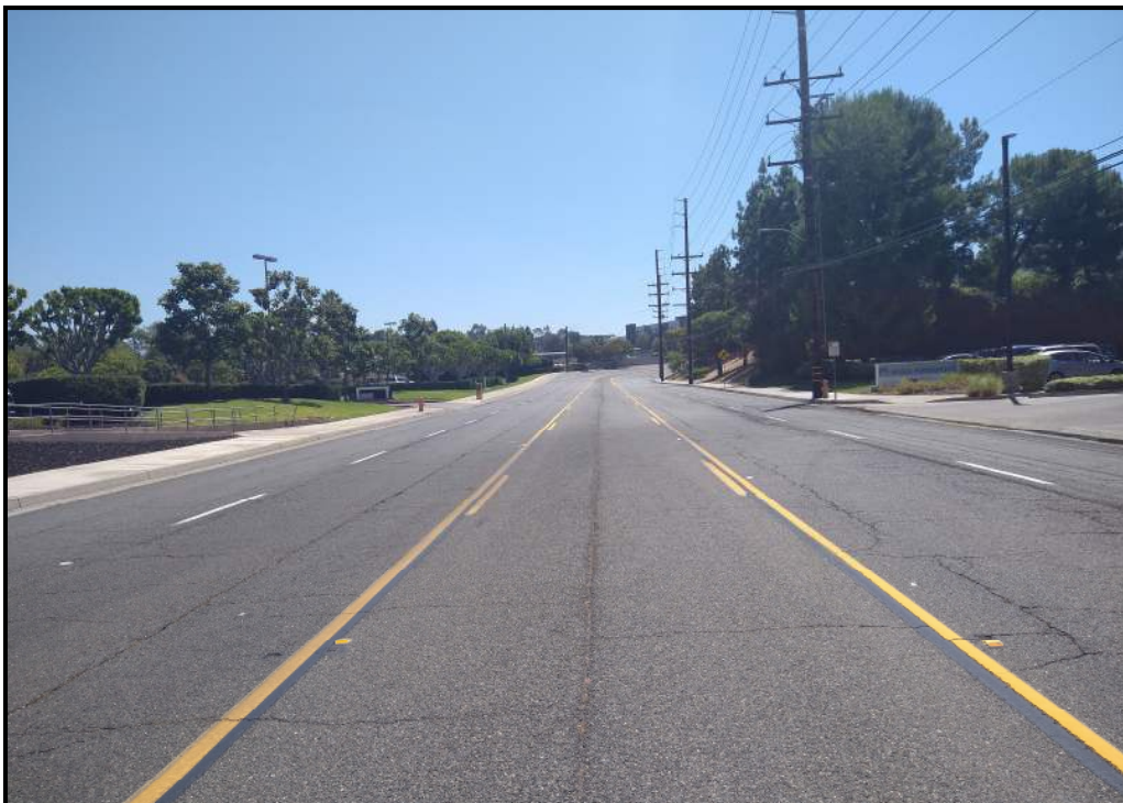
AVENIDA DE LA CARLOTA ( Looking Eastbound ) at 23041 Office Building
