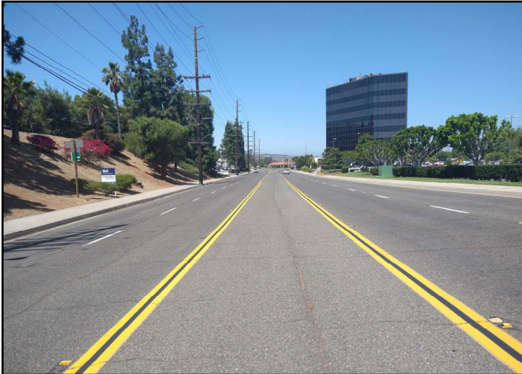
AVENIDA DE LA CARLOTA ( Looking Westbound ) from Curve Approx. 1,000 Feet East
