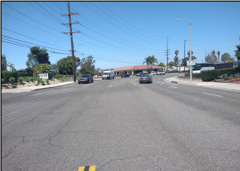
AVENIDA DE LA CARLOTA ( Looking Westbound ) from Plaza Pointe Drive
