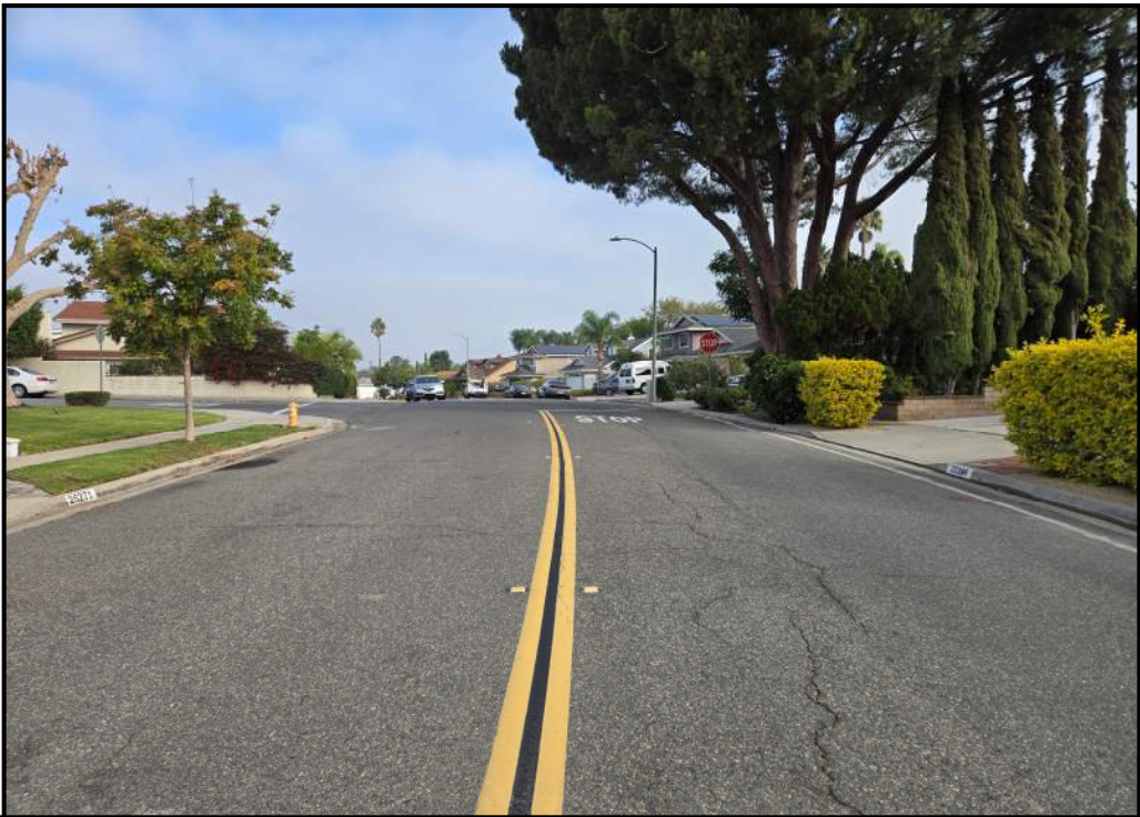
ERICSON WAY (Looking Northbound) at Earhart Road (south)
