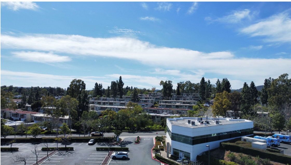
Image 2 - 65 ft. at Mill Creek showing the view of a building with existing height limitations
