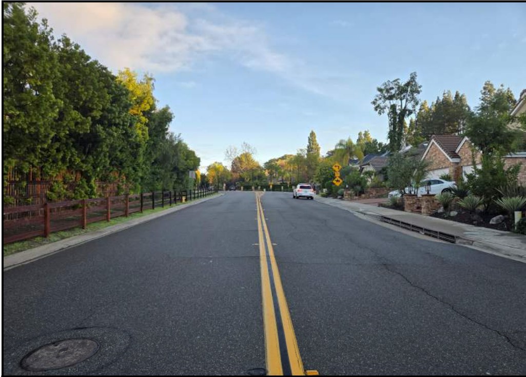
GREENFIELD DRIVE (Looking Northbound) towards the Northerly Equestrian Crossing
