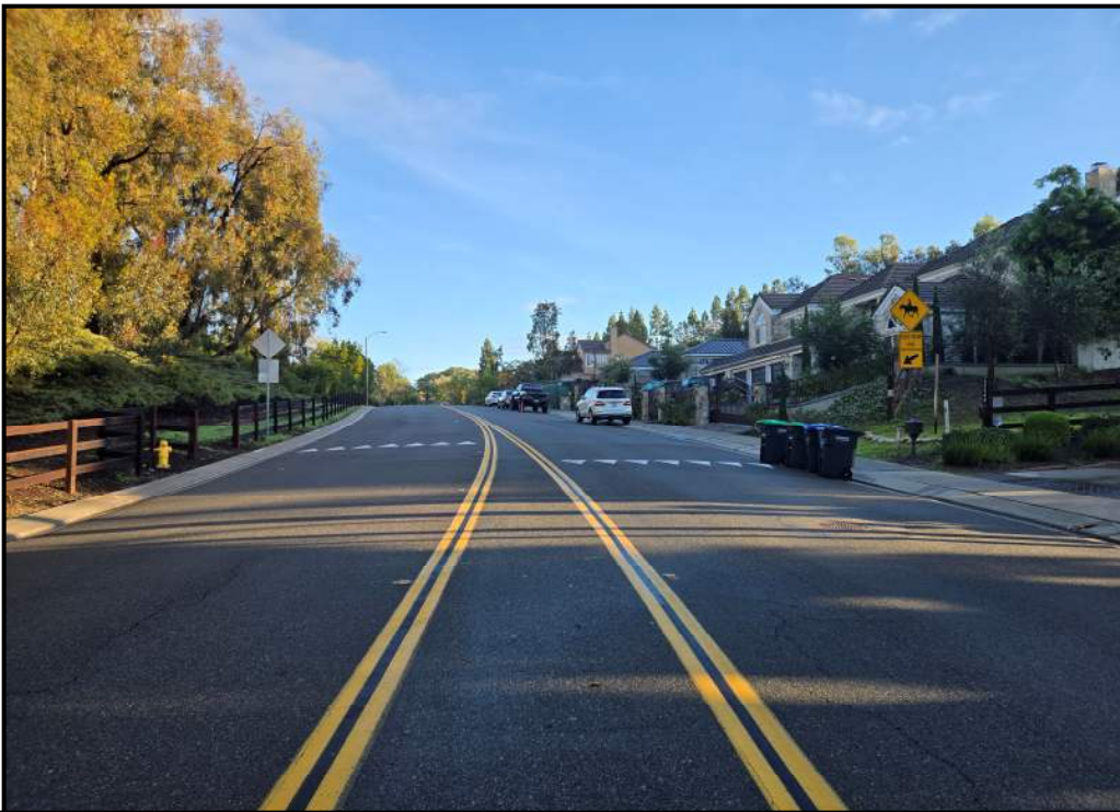
GREENFIELD DRIVE ( Looking Northbound ) towards the Southerly Equestrian Crossing
