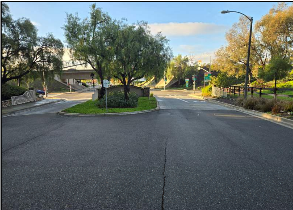
GREENFIELD DRIVE (Looking Southbound) towards the SR-73 Freeway
