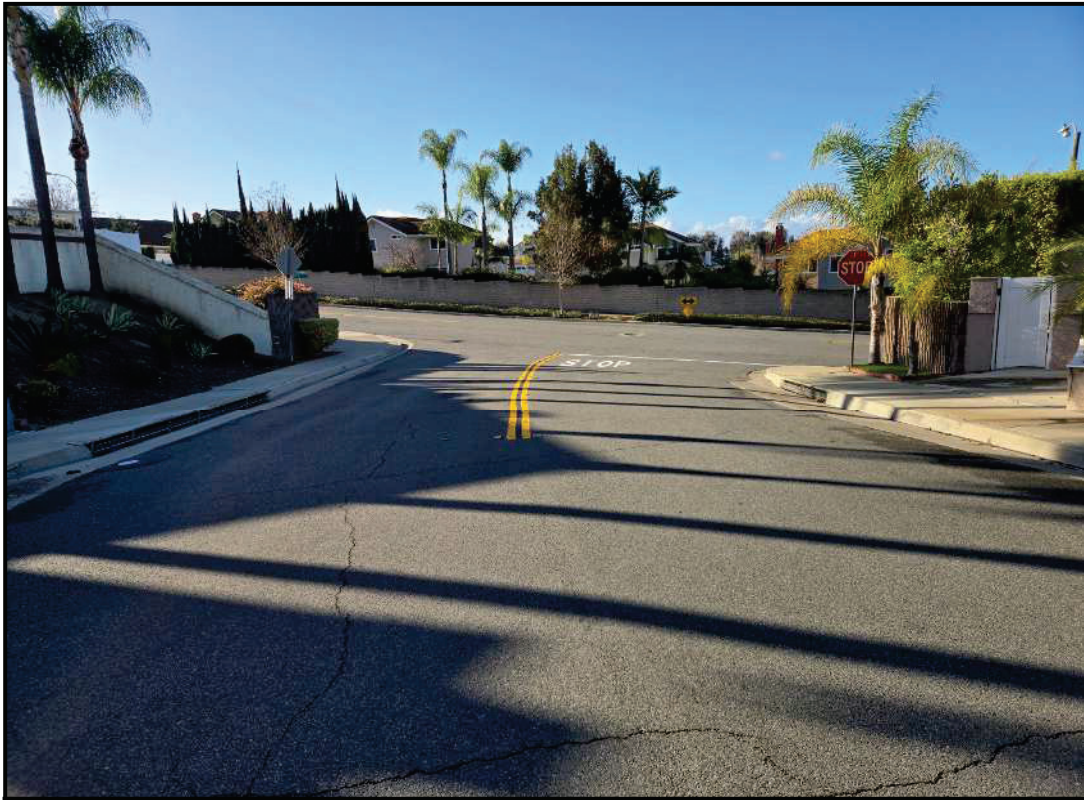
LA CIENEGA STREET ( Looking Northbound ) at ALISO HILLS DRIVE
