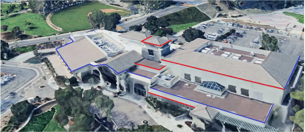
Aerial view — highlighted roofline segments for C9 lighting placement
