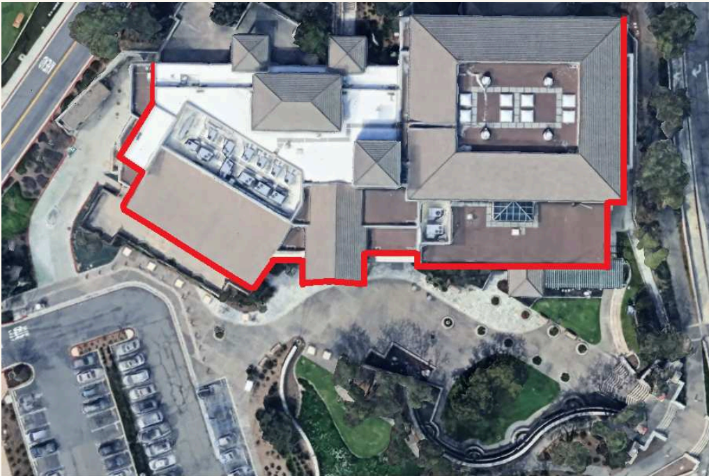
Overhead view — full roofline lighting path, highlighted in red
