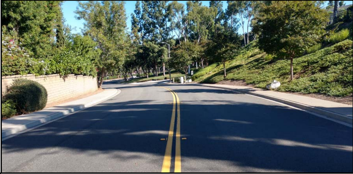
SANTA VITTORIA DRIVE (Looking Northbound) @ SAN REMO DRIVE
