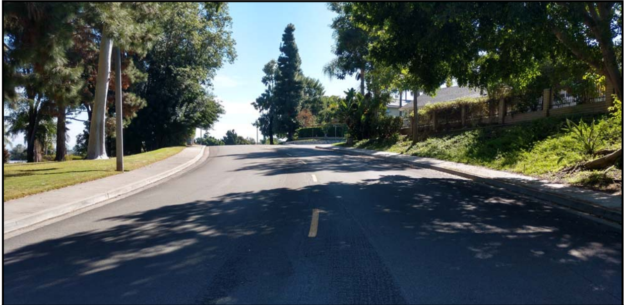
San Remo Drive (Looking Eastbound) at Pesaro
