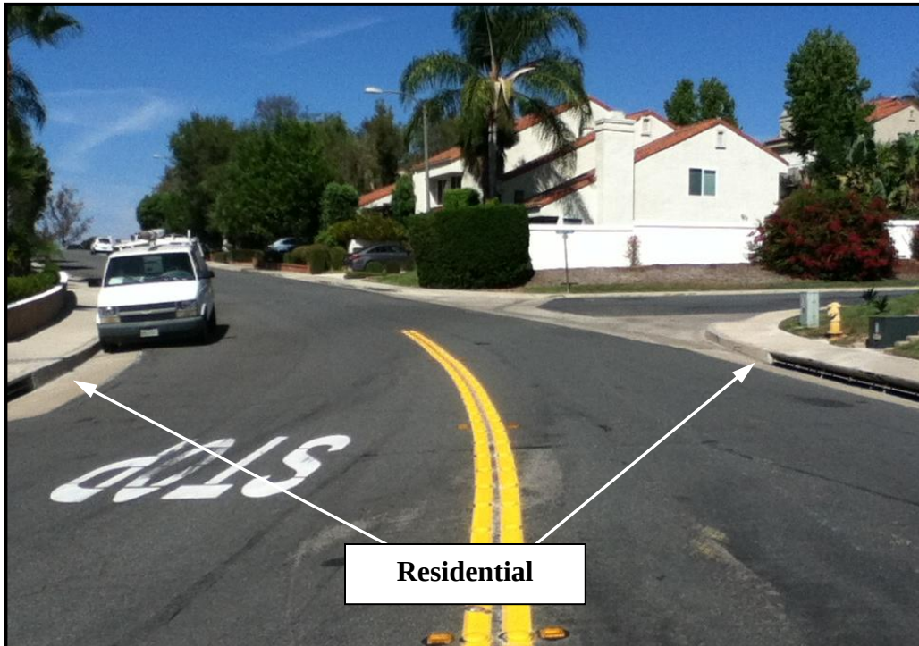
EL SEGUNDO STREET (LOOKING NORTHBOUND) @ LINDA FLORA STREET
