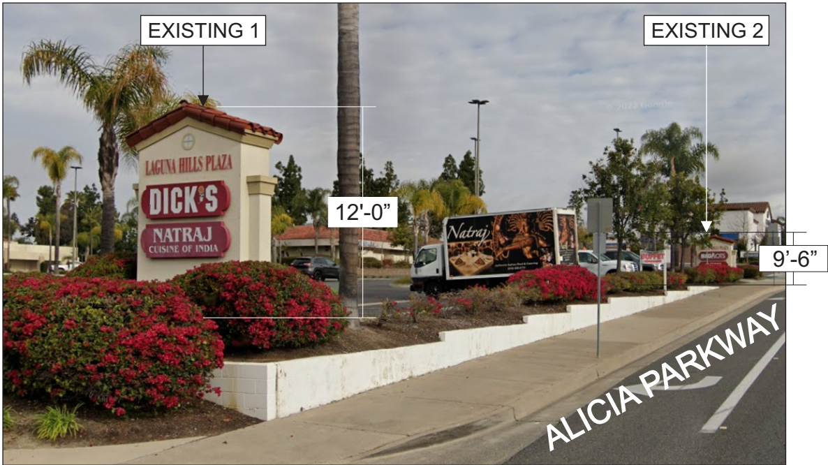
EXISTING CONDITIONS - SIGNS TO BE REPLACED
