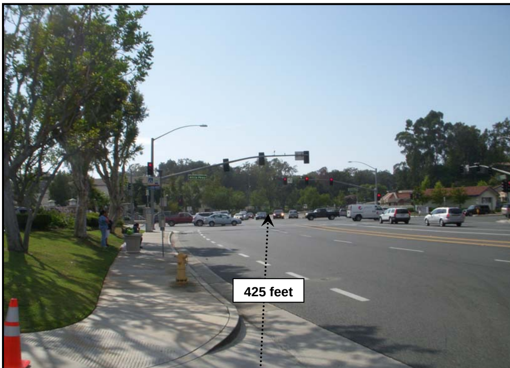
RALPH'S DW (LOOKING WEST) @ EB PASEO DE VALENCIA (DESIGN SPEED OF 50 MPH)
