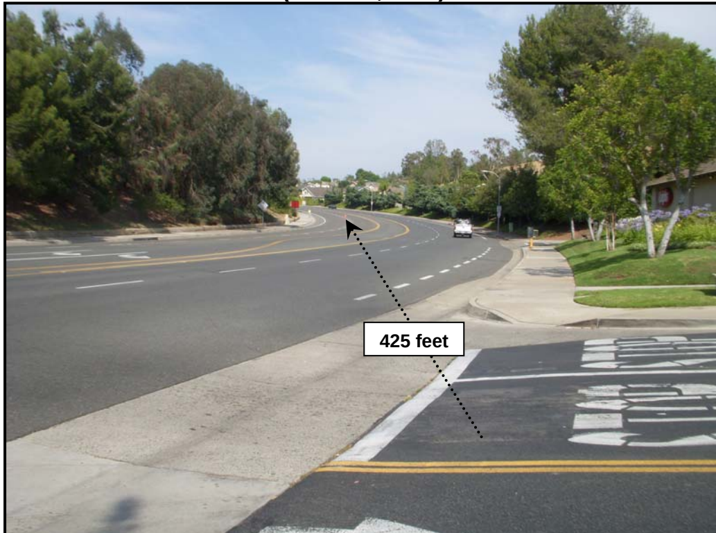
RALPH'S DW (LOOKING EAST) @ WB PASEO DE VALENCIA (DESIGN SPEED OF 50 MPH)
