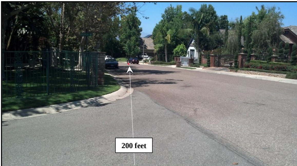
BROKEN BIT LANE (SOUTH-SIDE - LOOKING WEST) @ BUCKSKIN DRIVE
