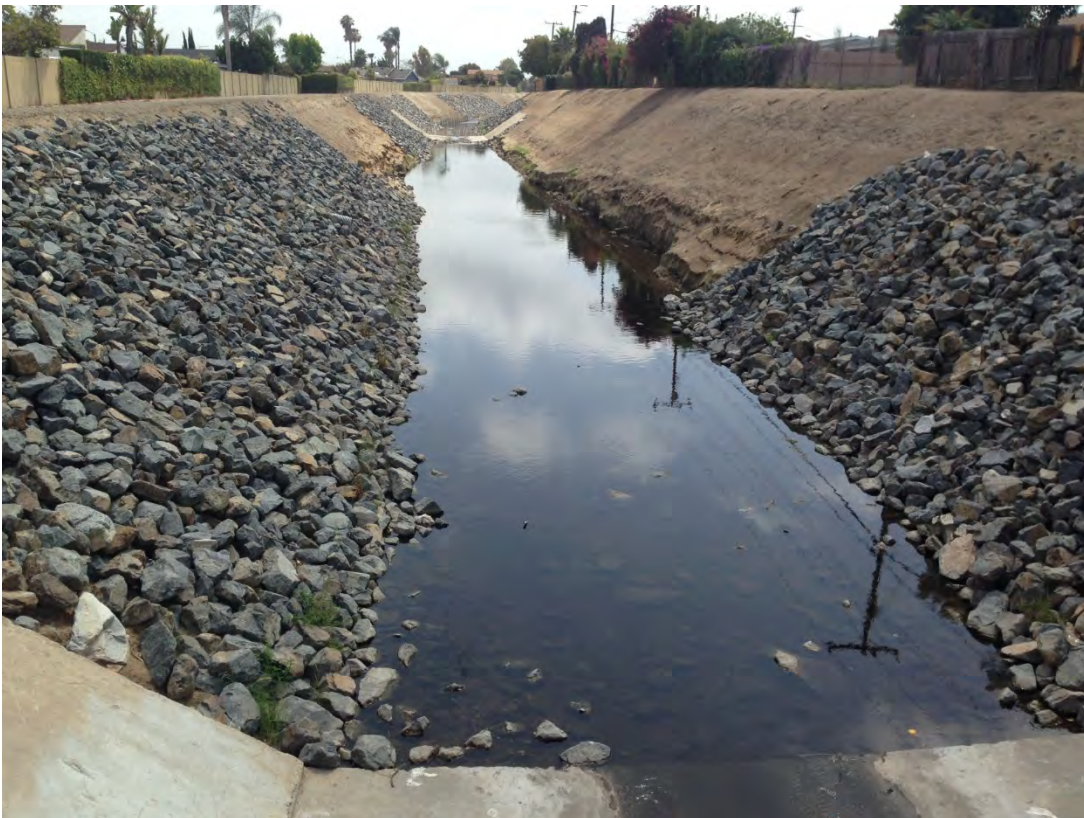
Photograph: Looking upstream at the Greenville-Banning Channel from the California Street bridge
