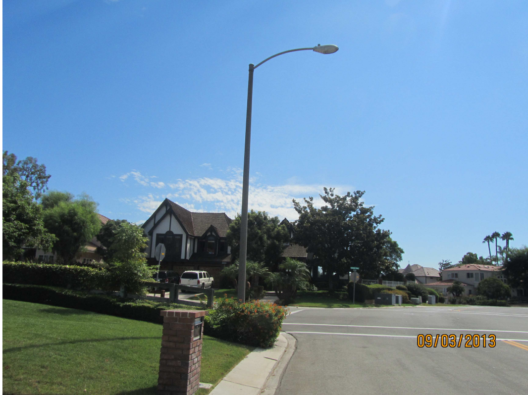
30' Mast Arm Street Light
