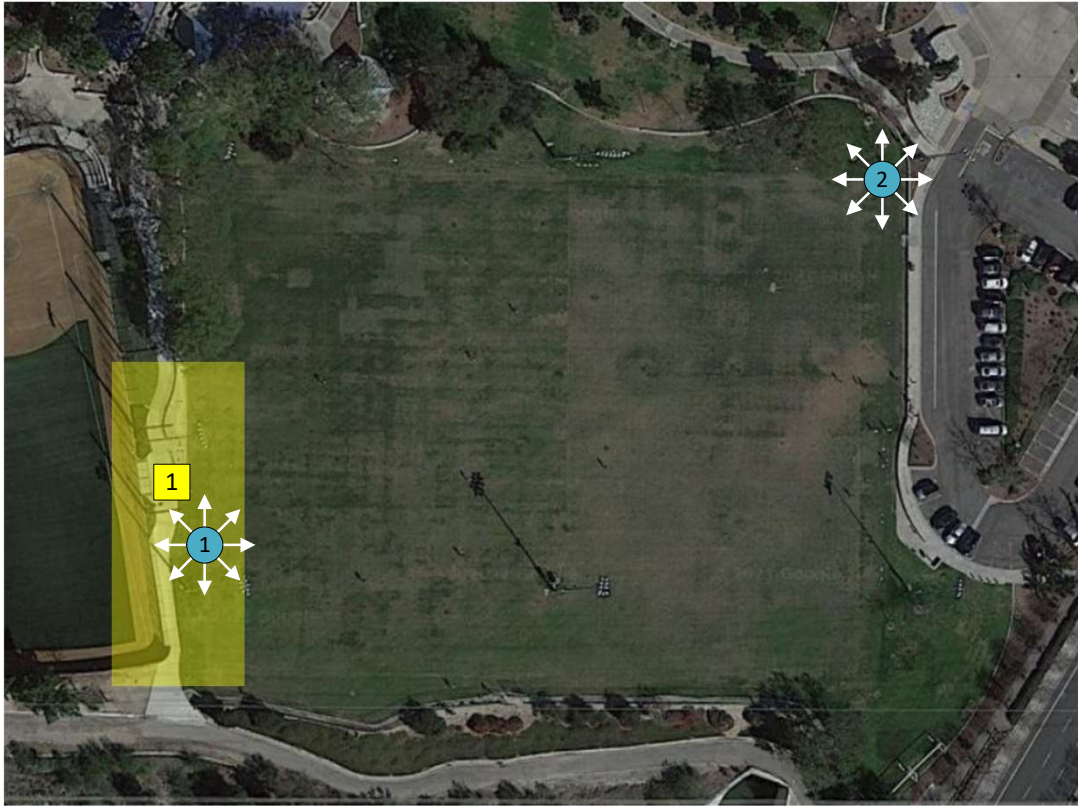
Light Pole Installation
