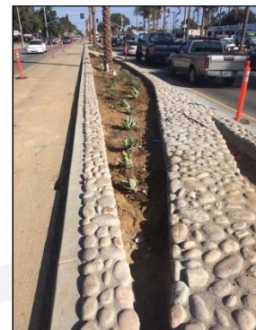
Newly landscaped median
