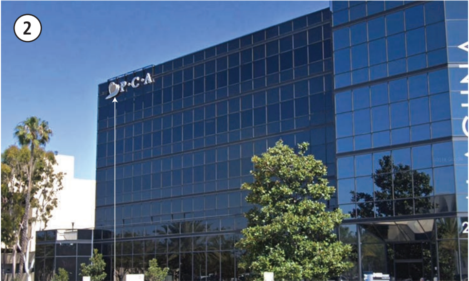
SIGN TYPE B.1: EXISTING FACE-LIT CHANNEL LETTERS ON 2" SQ. TUBE FRAME TOTAL SIGN AREA: 124.78 SQ. SF. (SEE SHT. #6 & 7 FOR LAYOUT & SPECS.)
