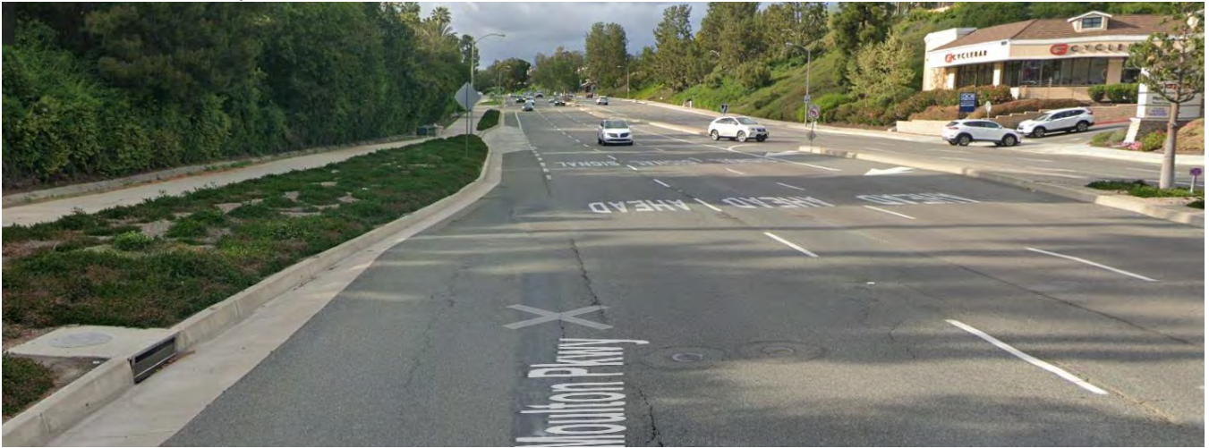
315 La Paz Rd 50' W/O Toll Road off Ramp S/S
