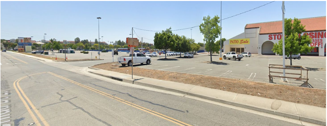
LH ID# 61 Avd Carlota 550' S/O Plaza Lane West Side
